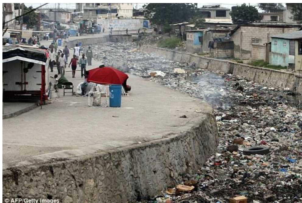
Figure 2. Drainage Canal – Downtown Port-au-Prince
